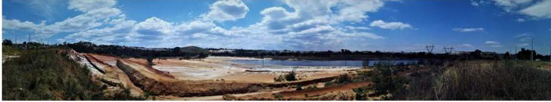
Lancaster dam in the above photo is classified as a Class F dam, and a radioactive hot spot. The re-mining of the tailings has caused this hazard. The only warning signs to the public are cardboard 'no entry' signs on thin wooden sticks that get blown over.
